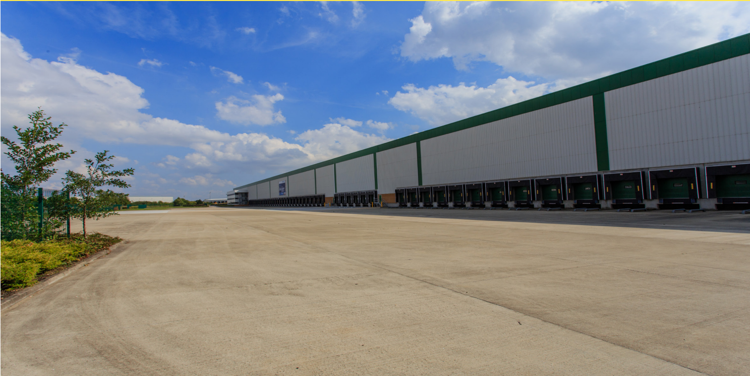
The Big 555 in Sherburn in Elmet where Logicor have leased the largest available warehouse in the UK, totalling 556,126 sq ft, to L&G Homes.
